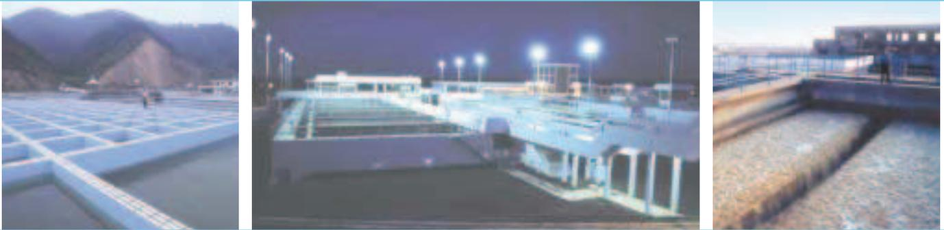
Designed for drinking water plants, Aquazur V is a descending current open sand filter. It retains suspended particulate matter in raw water thanks to a thick layer of sand. The homogeneity of the sand increases the filter run time, while the thickness enables filtration at high speeds and the high water head (1.20 m) prevents degasification.
